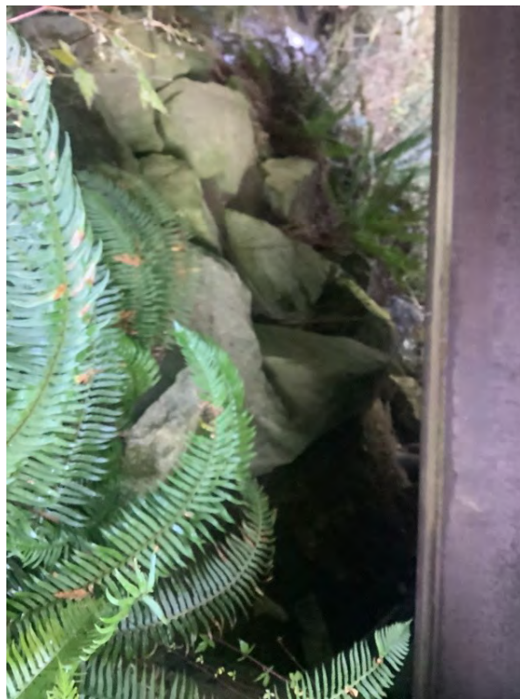
Right Bank Abutment when facing downstream
