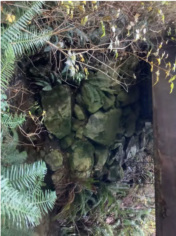
Left Bank Abutment when facing downstream
